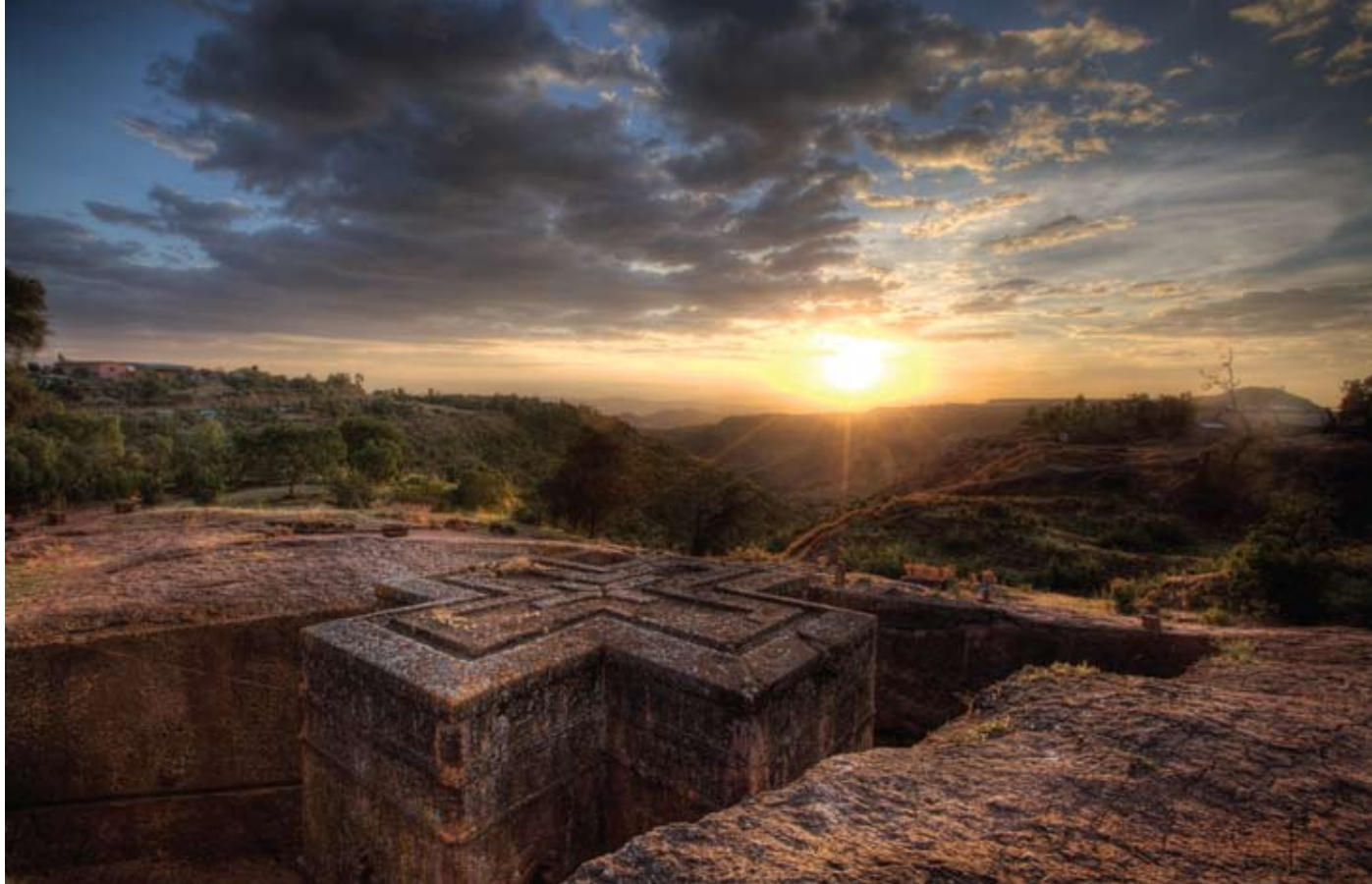
Lalibela, Ethiopia. St. George church. This church is carved out of solid rock and one has to walk down a path that descends 100-feet to get to the entrance. The insides of the church are similarly carved out from the same rock.
